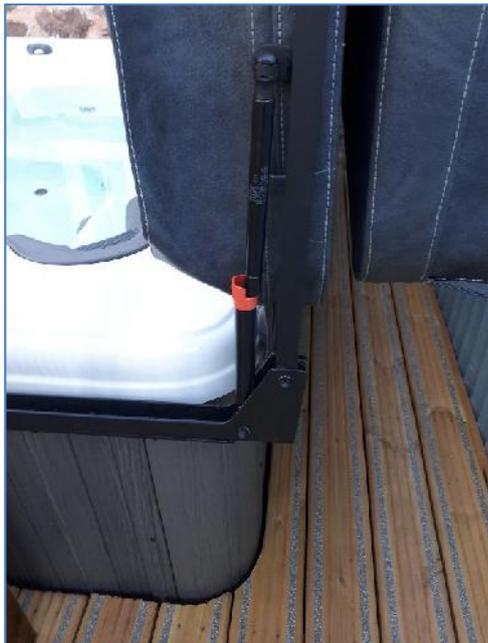
**Photo 2:** To close, press red catch in and push across to allow the black strut to line up and drop into place
